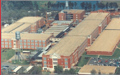
B.F. Goodrich Building - Thomaston, Upson County
