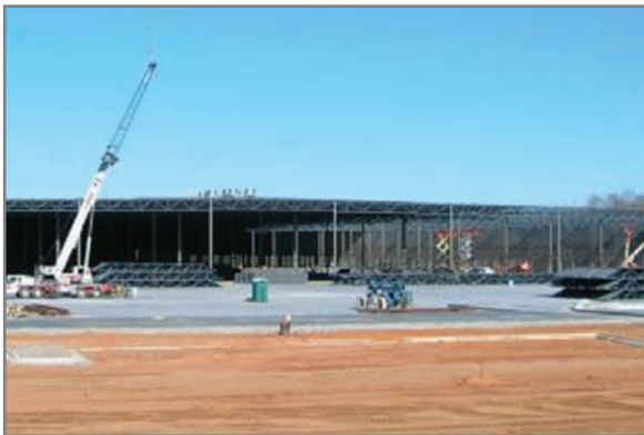
A 960,000 square-foot building in Commerce I-85 Business Park is under construction.
